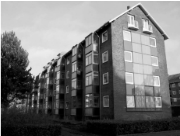
Figure 16 House end with solar mass wall. West facing glazed balconies
