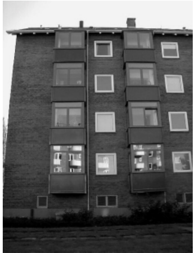
Figure 18 Glazed balconies with ventilated solar walls in parapets
