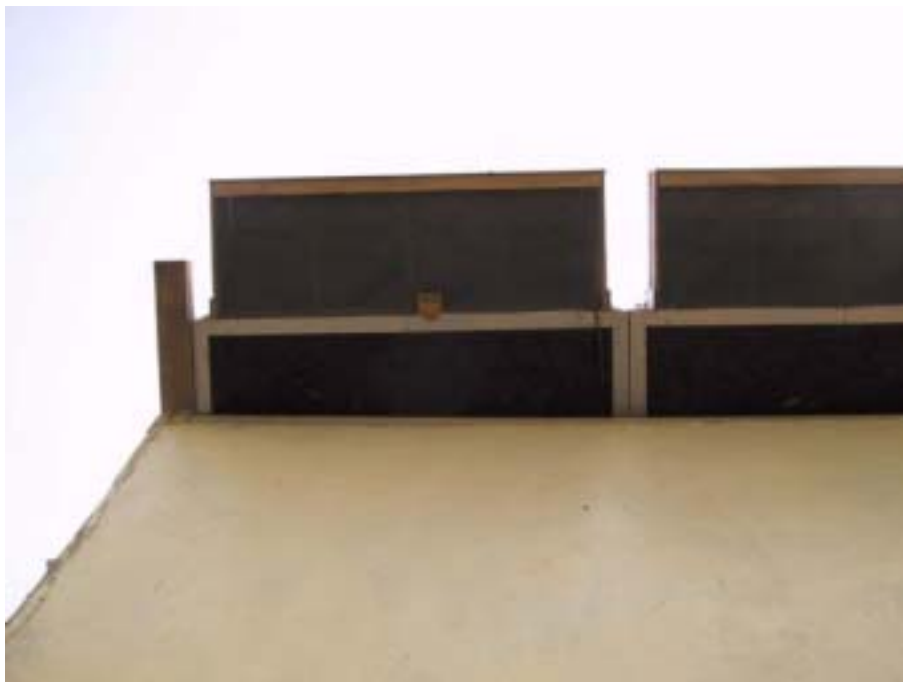
Figure 2.13. The combined temperature/humidity sensor at the top inlet to the solar air collector.
