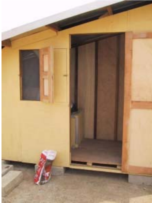
Figure 3.2. The solar fish dryer seen from the east. The dryer has two hatches in the east wall with insect net and an entrance door.
