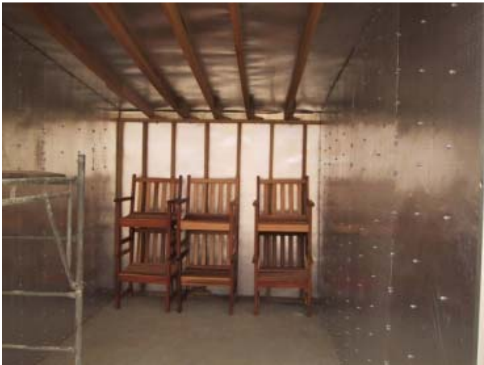
Figure 4.7. The chamber of the solar kiln before the false ceiling and fans were installed.
