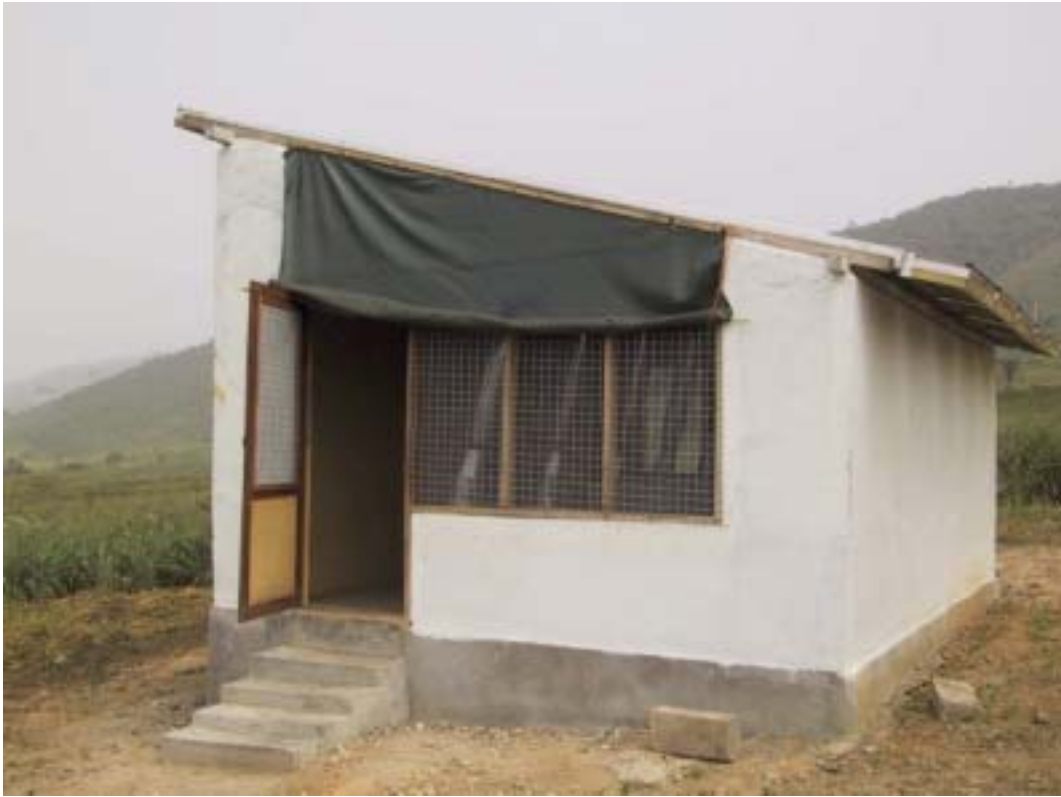
Figure 2.3. The solar crop dryer seen from the west.
