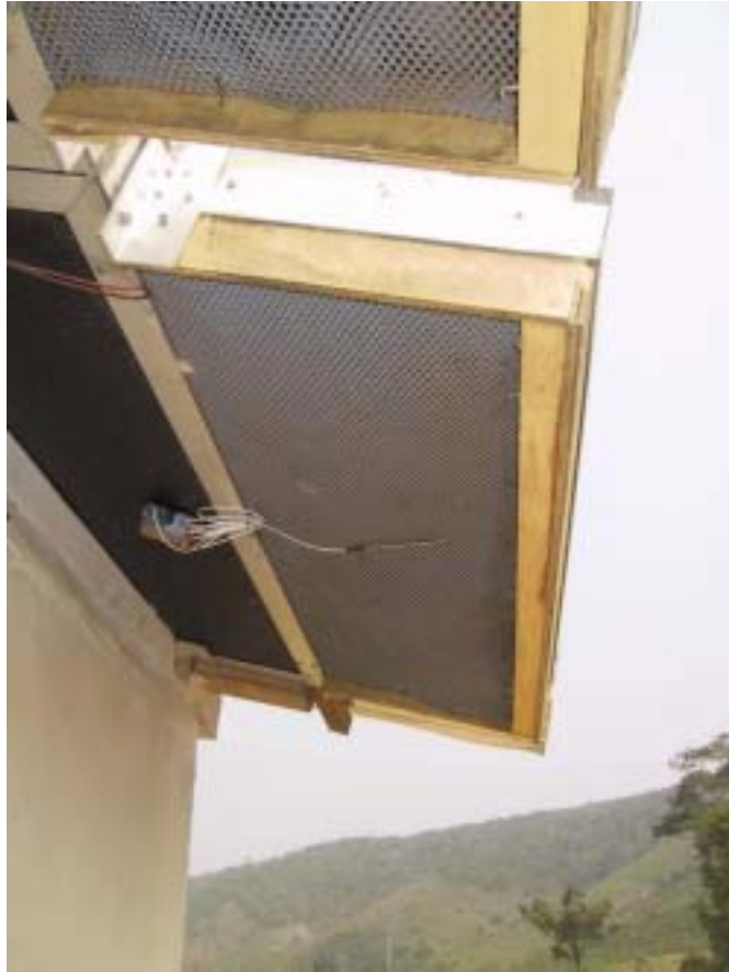
Figure 2.16. The temperature sensor at the bottom inlet to the solar air collector.
