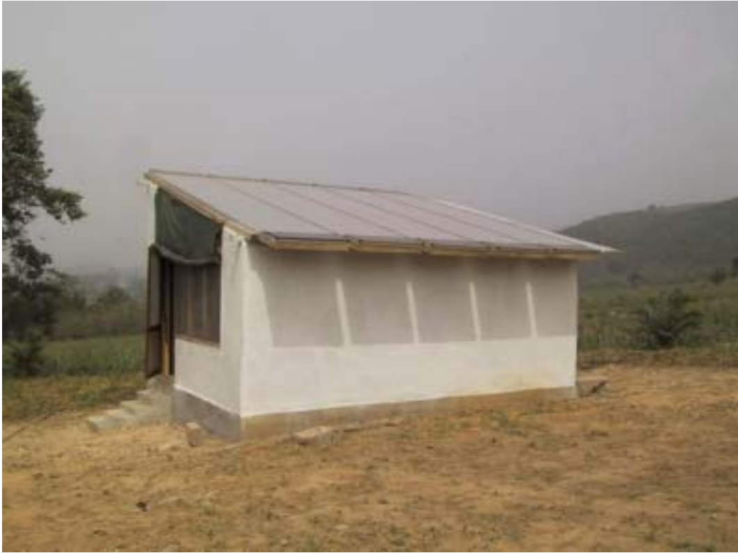
Figure 2.2. The solar crop dryer seen from the south.
