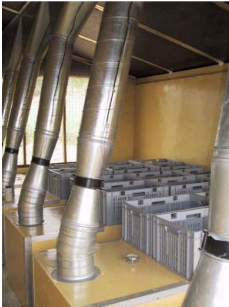
Figure 2.4. The five drying units inside the building.
