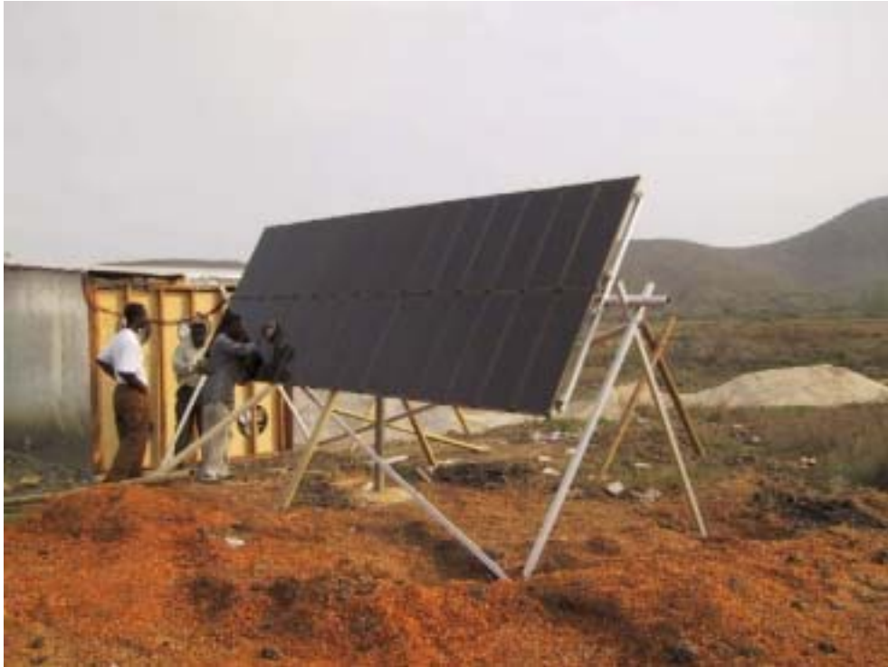
Figure 4.5. The PV-panel turned to face west – being cleaned.
