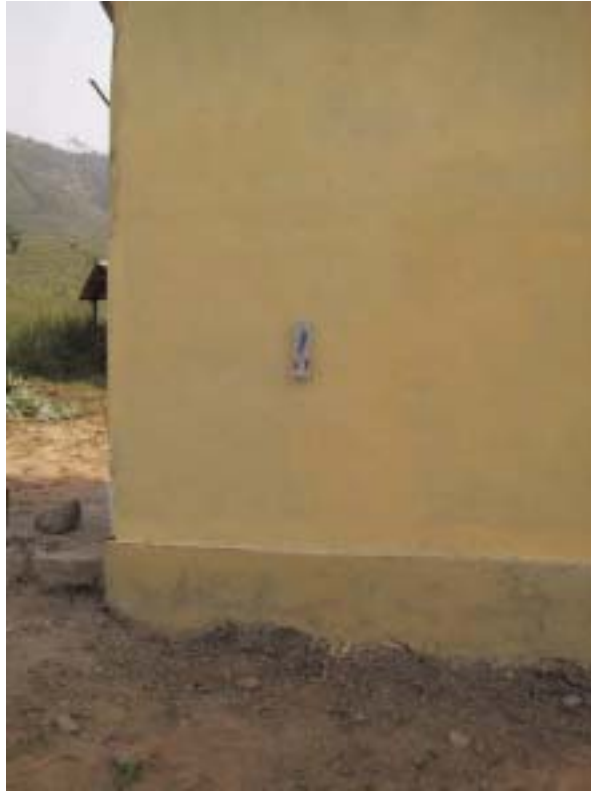
Figure 2.9. The location of the Kreiberg psychrometer for measuring of ambient temperature and relative humidity at the north wall of the building.
