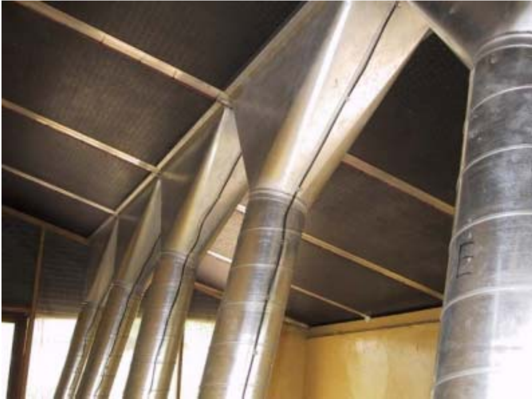
Figure 2.5. The connecting ductwork between the solar collectors and the drying beds.
