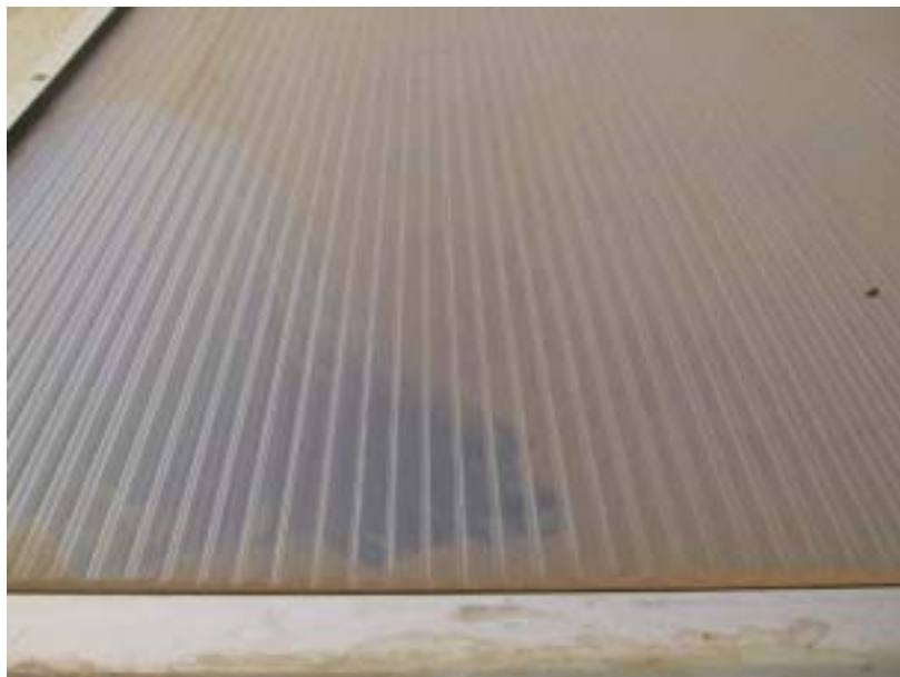
Figure 3.6. Dirt on the solar air collector – the PV-panels (not shown here) had been cleaned the day before, but already rather dirty.
