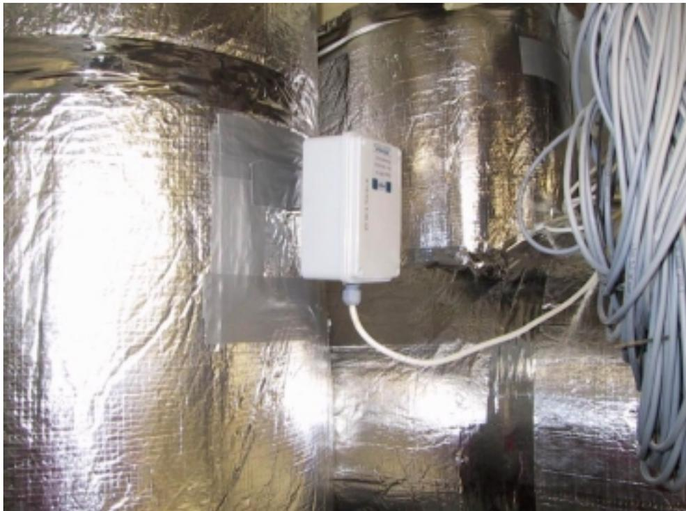
Figure 3.8. The applied Envic type AFT-10 air speed sensor in the exhaust duct.
