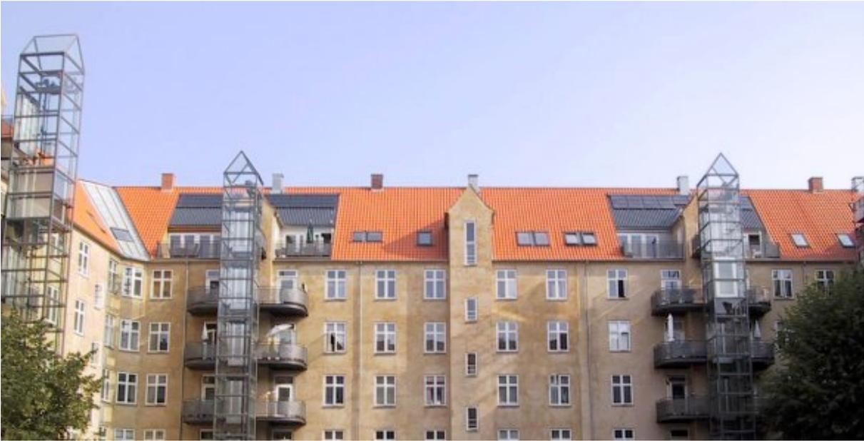
Figure 1.3. The two PV/solar air collectors mounted on the roof above two staircases.
