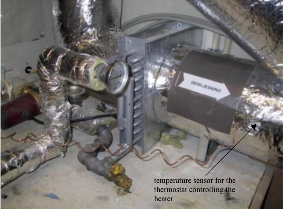
Figure 2.19. The heater after one of the small heat exchangers.
