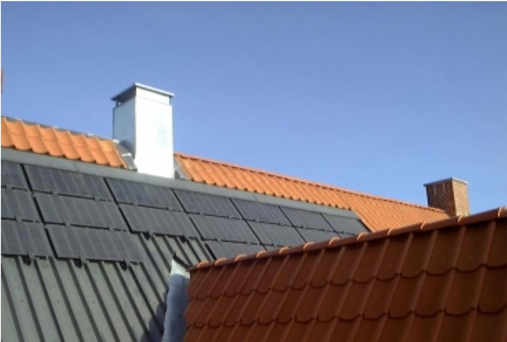
Figure 1.4. Close up of one of the PV/solar air collectors.
