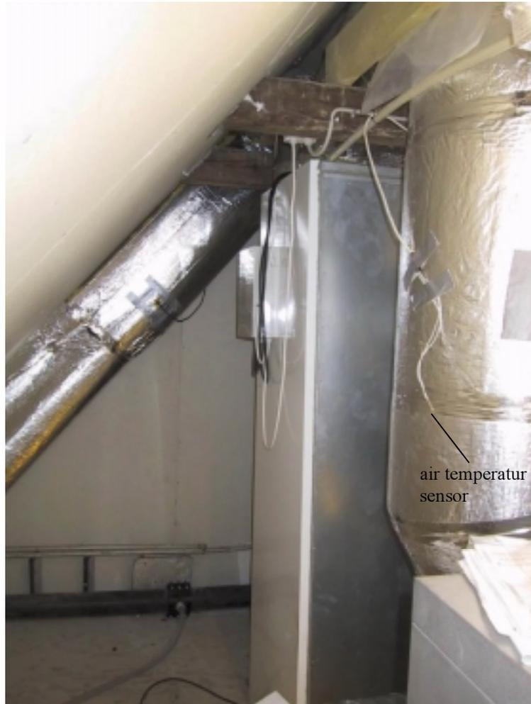
Figure 3.9. The temperature sensor measuring the air temperature in the technician room.
