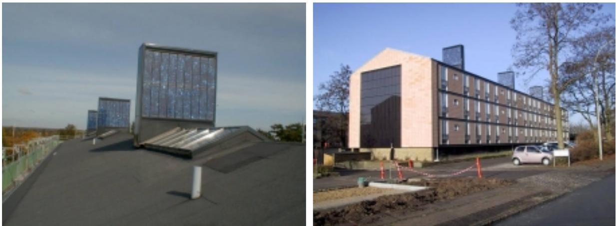
Figure 4.32. The solar chimneys at Lundebjerg for which the efficiency curve in figure 4.31 was found.
