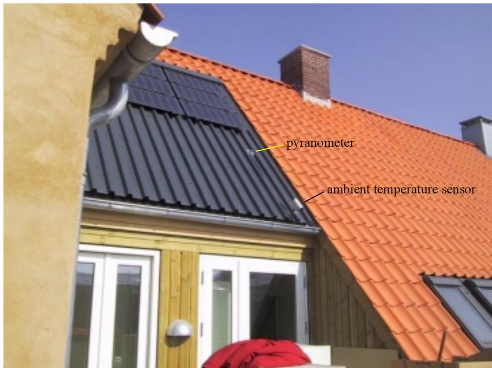
Figure 3.1. The pyranometer and ambient temperature sensor
