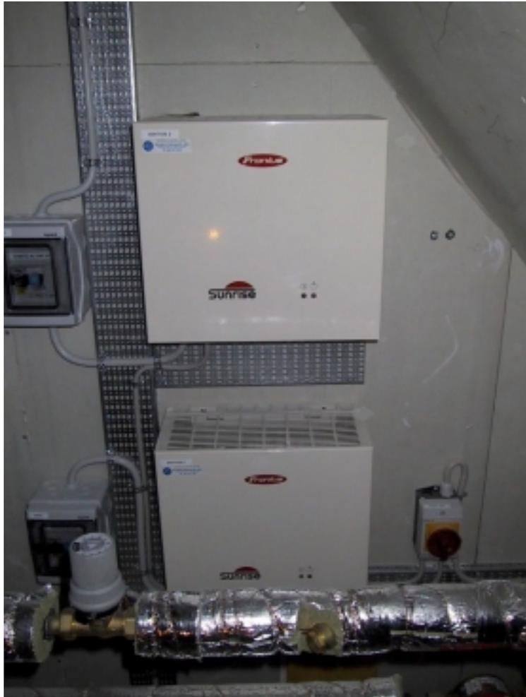
Figure 2.11. The two Sunrise inverters – one inverter for each of the two PV array.
