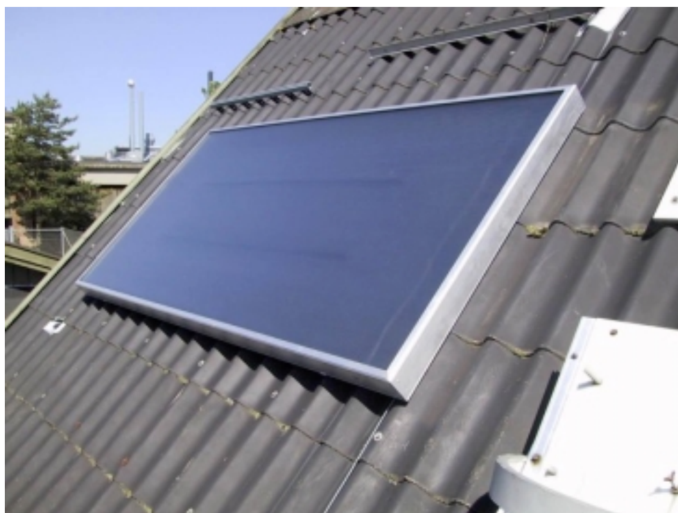
Figure 2.17. The single solar air collector with fibre cloth absorber mounted at the roof of the laboratory of Solar Energy Centre Denmark, Danish Technological Institute.
