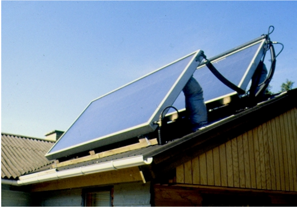
Figure 1.2. Example of two hybrid solar air/liquid collectors (solar air collectors where liquid is circulated in the absorber) connected by means of ducts.
