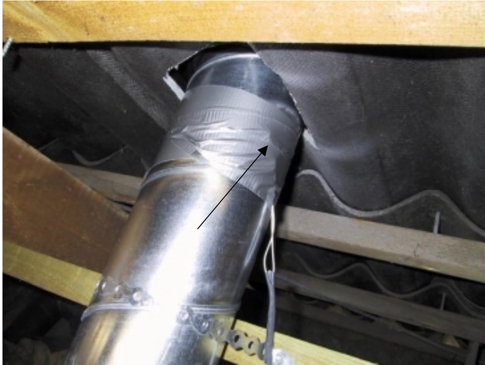
Figure 3.8. Location of the outlet temperature sensor for the single solar air collector with fibre cloth absorber.
